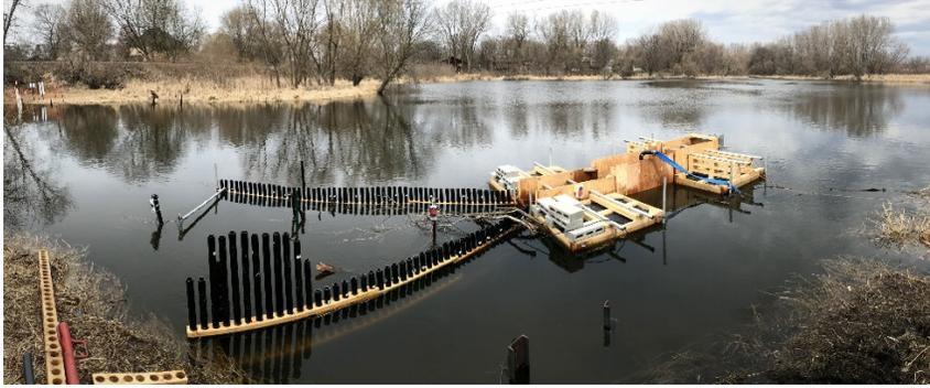
Kukulski — along with post-doctoral student Peter Hundt and University of Minnesota technicians Kao Vang and Cameron Swanson — pounded black PVC pipes into a collar that will hold the repositioned chute in place.
