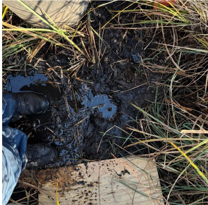
Figure 1. Wet conditions observed during October 18, 2024, Visit
