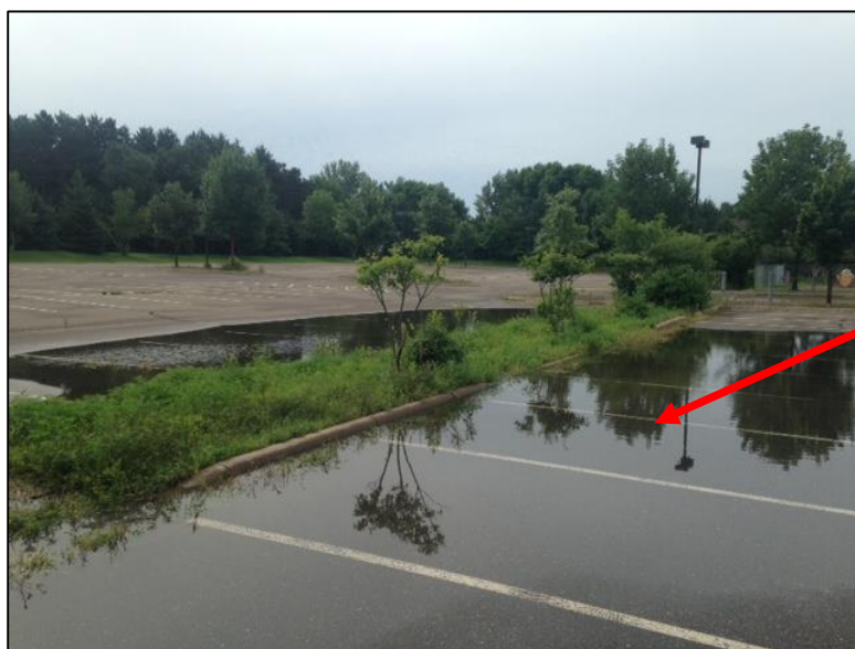
Figure 20. Flooding at Site 6 (left) in the Pleasant catchment (August 2015), Incarnation Lutheran Church parking lot. The proposed BMP involves removing some parking spaces to expand the vegetated area, creating a raingarden to which most of the back parking lot drains. (Right). Map of bioretention sites 1-6, Pleasant Catchment.
