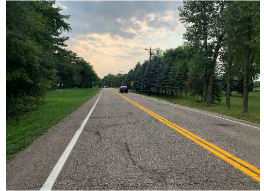
Figure 17: Ash Street (Anoka County)
