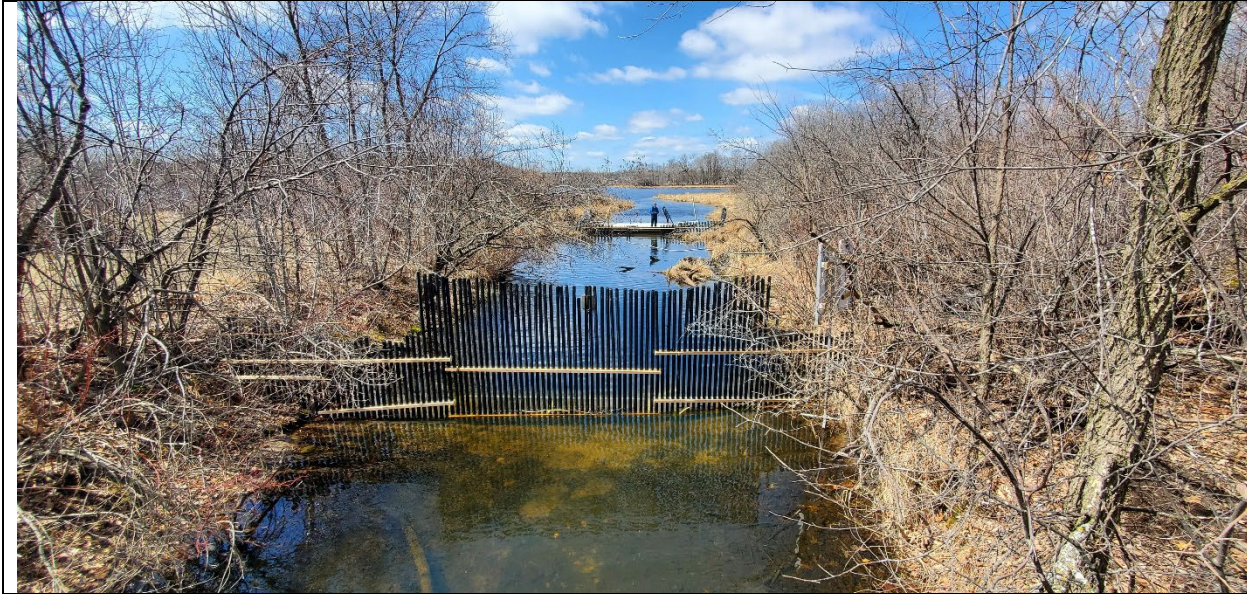
Carp stream removal preparation
