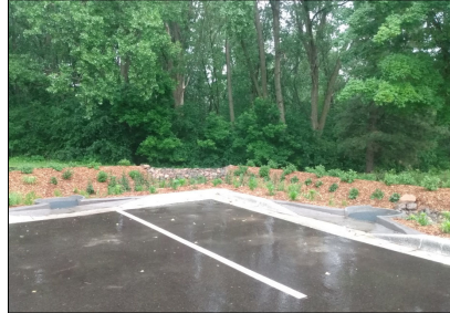
Create new storage Bridgewood Rain garden
