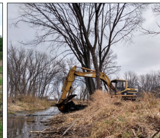
Maintain existing infrastructure Lambert Creek Dredging
