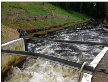
Repair infrastructure Koehler Road Bank Restoration
