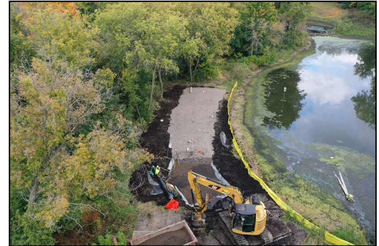
Above: The Whitaker Pond Biochar Filter pictured during construction in October 2022.
