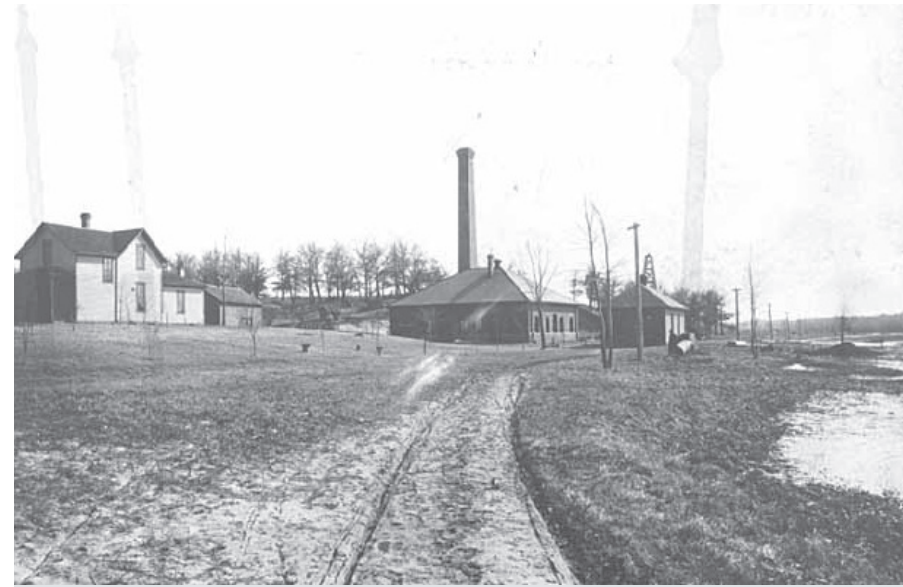
Vadnais Lake pumping house, early 1900s - courtesy of MN Historical Society
