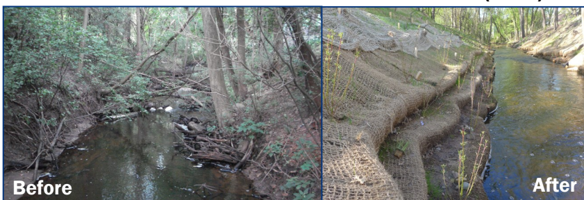
Lambert Creek bank restoration at Kohler Road (2017)
