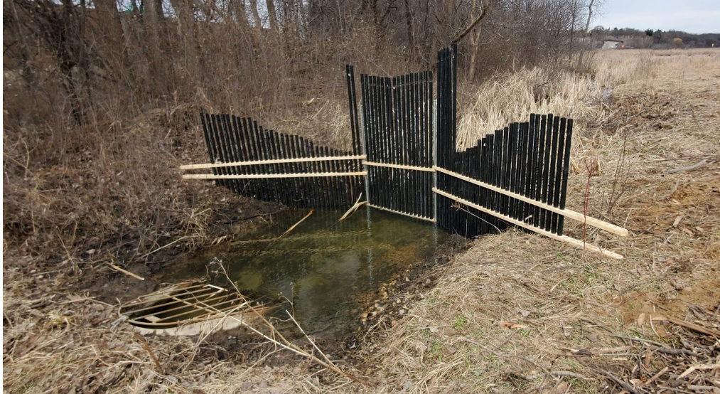
Figure 2: Picture of the physical barrier at the outlet of West Vadnais
