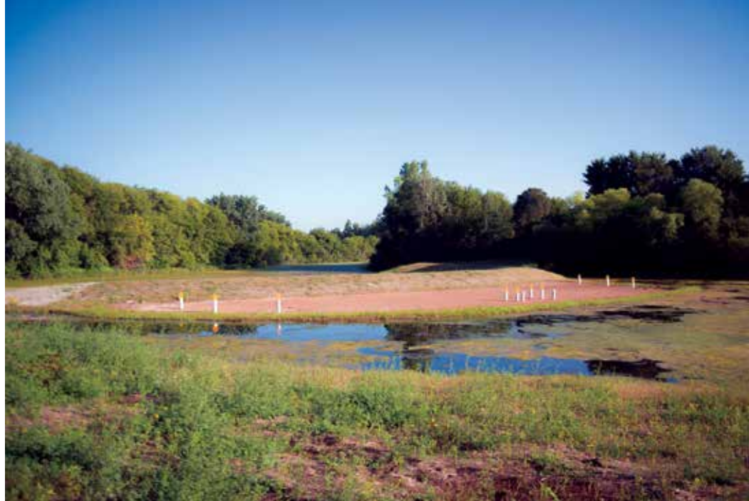
Figure 4. An iron-enhanced stormwater filter on a key stormwater pond draining to Bur Oaks Lake in Eagan, MN. Designed by Wenck Associates, Inc. Photo: Joe Bischoff.
